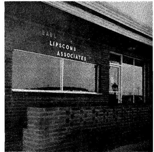
Houston Branch Office
